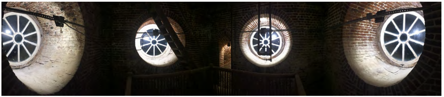
ROB & DAWN MCCREADY HAVE GENEROUSLY WORKED TO REILLUMINATE THE BELL TOWER AND STAINED GLASS IN THE SANCTUARY
